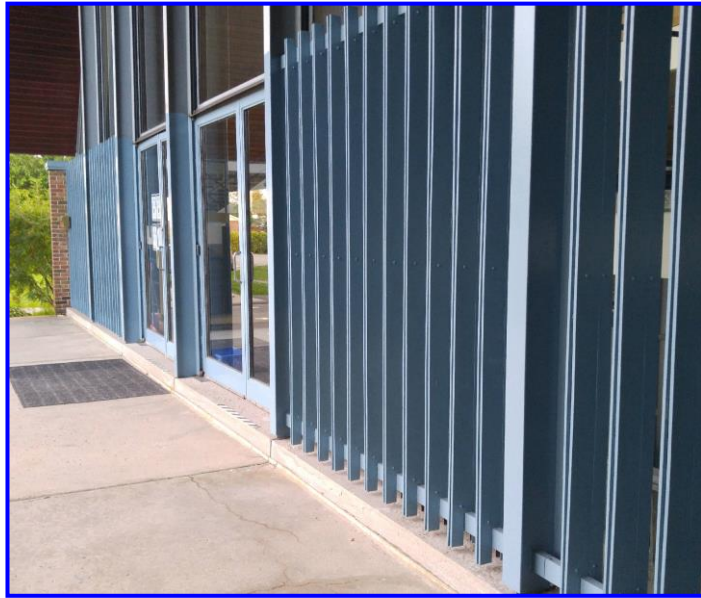
Newly painted church entrance
